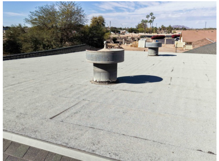
Installing a fully-adhered, reinforced elastomeric membrane over the existing cap sheet.
