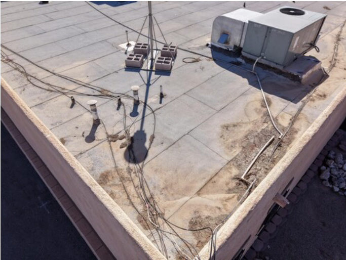
Reinforce drain perimeters and scuppers using mastic and fabric to prevent ponding or water intrusion.
