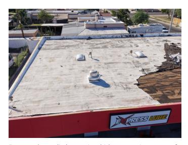
Foam can be applied at varying thicknesses to improve roof slope, directing water toward drains and preventing ponding water.
