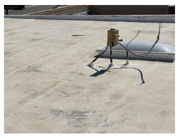
Electrical boxes will be disconnected, sealed, and properly covered to maintain roof integrity and prevent moisture intrusion.
