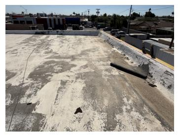
Clean and clear all roof drains to restore proper flow and eliminate standing water, ensuring the roof drains efficiently after rainfall.
