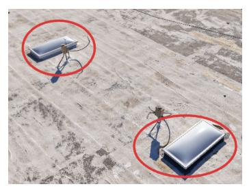
Two existing skylights will be cancelled and removed. The openings will be securely covered with new decking and integrated into the foam roofing system to create a smooth, watertight finish.
