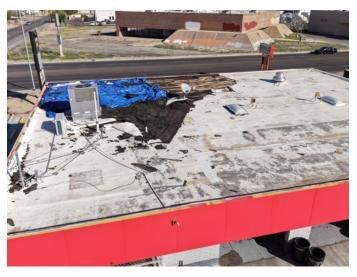
All existing roofing materials will be removed down to the deck to ensure proper preparation and optimal adhesion of the new spray foam system
