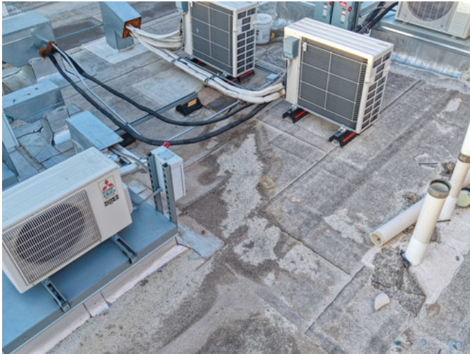
Clearing all loose materials from the roof surface.
