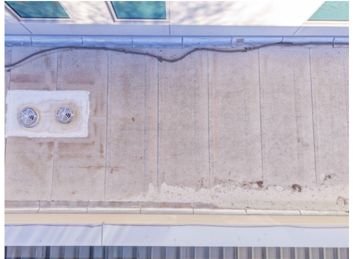
Seal and reinforce all mechanical curbs with high-build flashing grade sealant.
