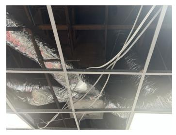
This photo shows the existing ductwork above the ceiling, with old flex runs and wiring exposed. The new duct system will replace these lines with properly sized, sealed, and supported flex ducts to improve airflow and efficiency.
