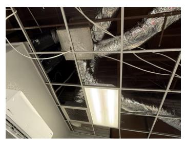
This photo shows the existing ductwork above the office area. The current setup has restricted airflow and uneven distribution. The new duct system will improve airflow, comfort, and efficiency, helping the unit run smoother.
